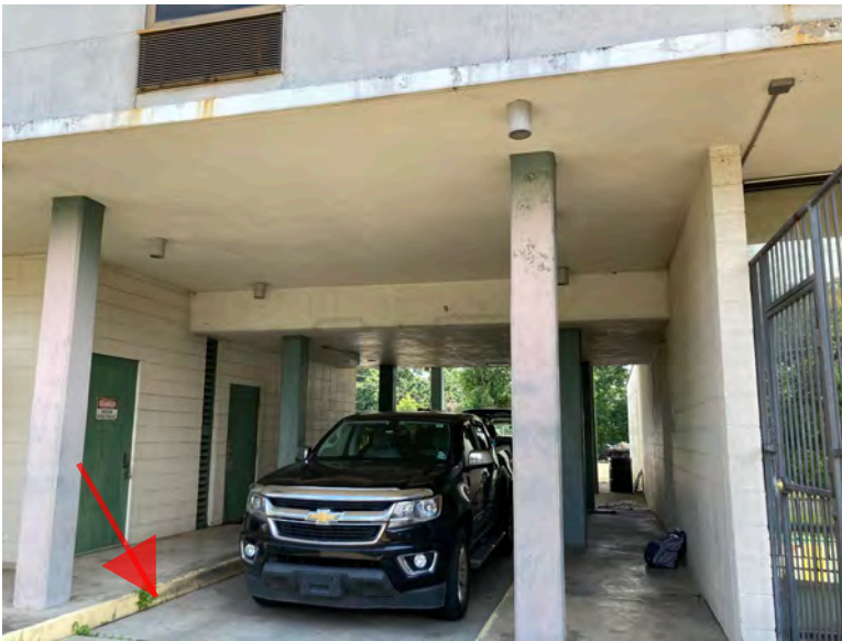
Exterior Concrete Curb (yellow)
