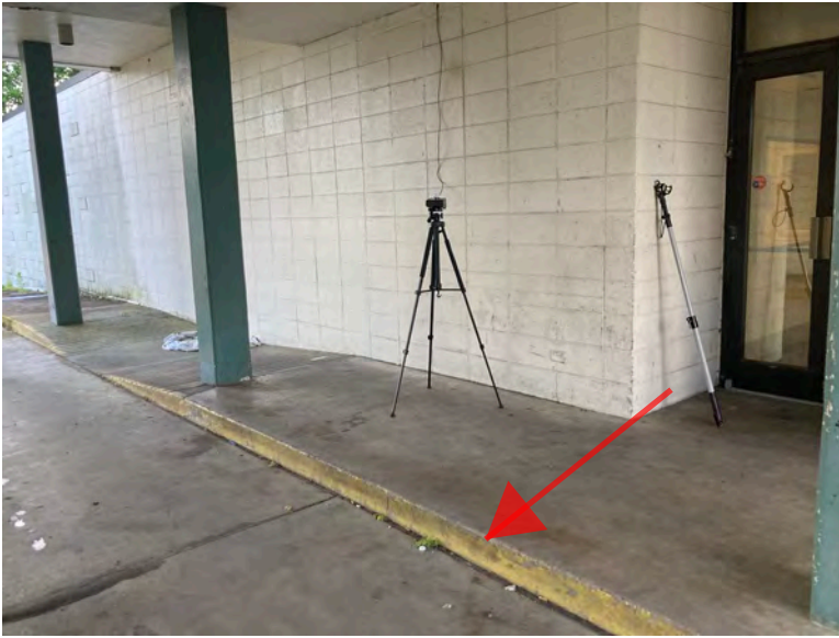
Exterior Concrete Curb (yellow)
