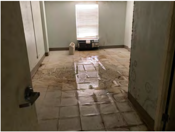
4 th Floor Room
