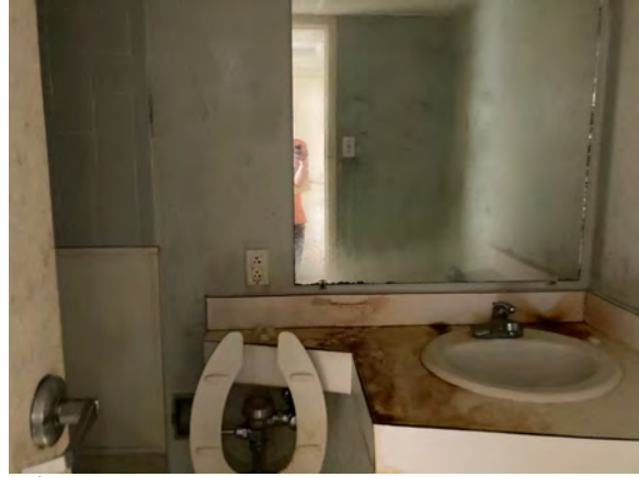
3 rd Floor Bathroom
